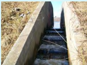
Fishway exit channel modifications
